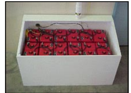
Deep-cycle batteries.
