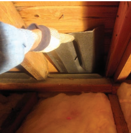
Place rafter vents in between the rafters where the ceiling meets the floor.
