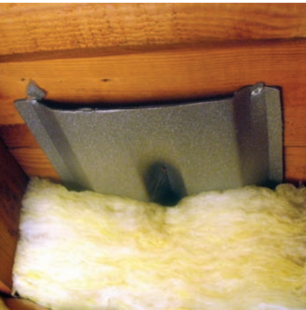
Add insulation around the rafter vent and out to the edge of the attic floor.
